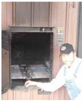
Edward Jewell says his new grate for Central Boiler wood furnaces is designed to burn wood more completely and results in less material to clean out.
