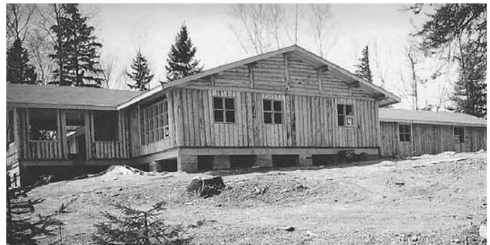
Vertical log homes use short 8 to 10-ft. logs that are easier to handle. The logs will also weather more effectively in a vertical position.
