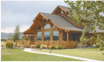
EverLogs are made of concrete, so living in an EverLog home means no worries about maintenance, log shrinkage, or insect damage.
