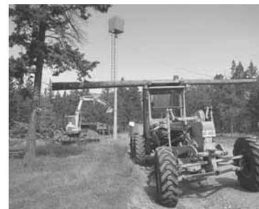
He chained a 30-ft. wooden pole down across the top of a road grader, then attached choker cables to both ends of the pole and pulled the tower up.
