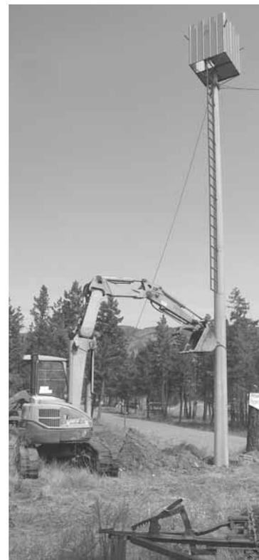
Errol Borsky's 45-ft. tall concrete tower has a cage at the top with enough room to fit 2 people comfortably. A ladder bolts to the top 24 ft. of the tower.
