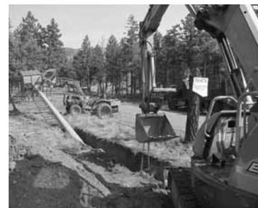
He used an excavator to dig a 7-ft. deep hole, then used a tractor equipped with a grapple fork to lift the pole into the hole.
