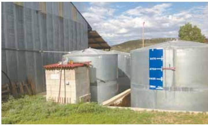
Dean Steward stores rainwater in tanks from multiple buildings on his farm. Pipes connect adjacent tanks. By installing mechanical gauges on the tanks, he can easily keep track of water levels.
