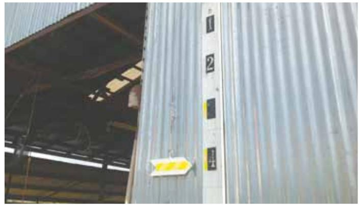
This gauge is mounted on a Quonset-style building. Aircraft cable runs from float in tank up over a pulley to a large pointer that moves up and down on scales of reflective numbers.
