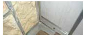
Panels are insulated with soy-based, closed cell foam.
