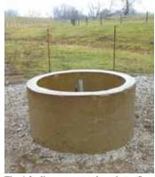
The 4-ft. dia. concrete culvert has a floor made of Quickcrete and is fed by an artesian well.
