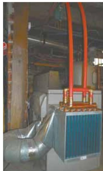
Matt Studer uses hot water from an outdoor wood burning stove to provide heat to his electric clothes dryer. He removed the dryer's heating element, then mounted a 12 by 14-in. plenum on one side. Two heat exchanger units, connected in series, attach to the plenum.
