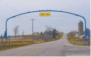
Chad Tasch uses a telehandler to set up his 20-piece "pipeline bridge" for liquid manure. Its end supports rest in roadside ditches, out of the way of passing traffic.
