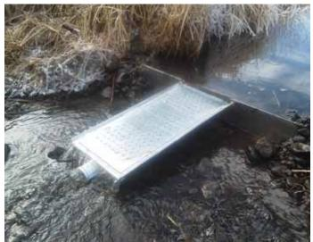
Water collection box "dams" the water in shallow streams, then pipes it to a cattle tank.
