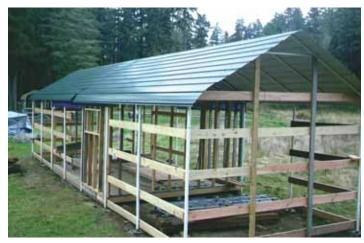
Stewart Kunkel used carport parts to provide the roof and frame for this 12 by 42-ft. Completed barn has plywood sides and a homemade gutter system. barn. Barn is shown here still under construction.
