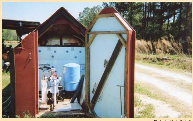
Entire back wall opens up for full access to well and pump.
