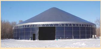
Project manager Paul Hofer reduced the slurry tank's 23-ft. high walls to 18 ft. and cut out holes for an entrance door and overhead door.
