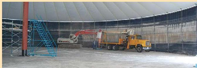
Inside, he installed a 50-ft. tall, 20-in. oilfield pipe at the center. A 5-ft. dia. steel frame is welded onto top of pipe.
