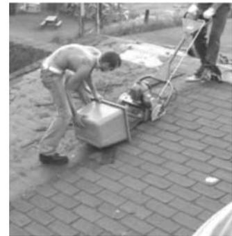
The Shingles Peeler picks up shingles, pulls out the nails, cuts the shingles, and then sends everything out back of machine.
