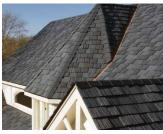
Made from recycled rubber tires, rubber "shingles" are a good alternative to expensive slate or shake roofing, says the manufacturer
