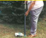
Just drop the spike down the pipe and drive it into the ground by pounding on the wood handle with a hammer. The spikes should be driven 2 in. below the surface, which is easy to do with this setup. (C.F. Marley, Nokomis, III.)
