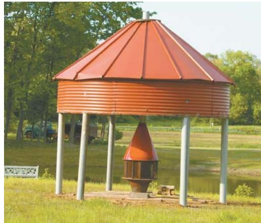
"Corn crib" gazebo has a free-standing fireplace in middle of floor, with a 6-in. dia. flue pipe running up through center of roof. Photo shows gazebo before it was enclosed with a wire fence grape arbor.
