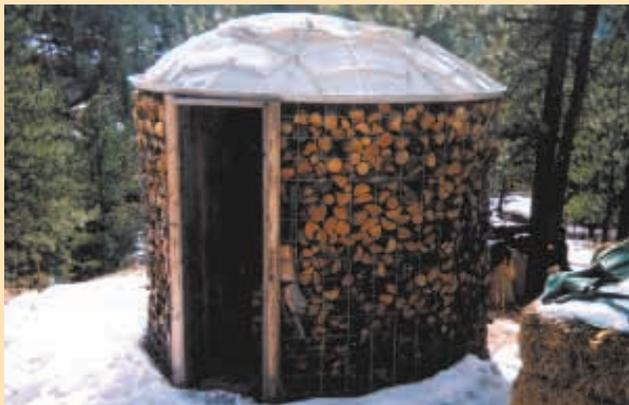
Jon Bell made use of an 11-ft. dia. satellite dish and a couple of cattle panels to make this wood shed. It holds six cords of wood.
