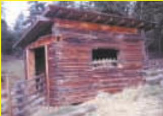
I built the walls on this horse shelter out of old mining core boxes. It measures about 10 ft. wide by 14 ft. long. The boxes are 10 in. wide by 5 ft. long and 2 1/2 in. high. I used a brad nailer to fasten the boxes together. It took only about four hours to build the walls. **(Gordon Fuller, P.O. Box 988, Barriere, B.C., Canada V0E 1E0 ph 250 672-0167)**
