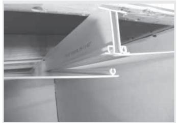
Zip-Up Ceiling Systems zip into place and zip back out when you need to work on plumbing or wiring.
