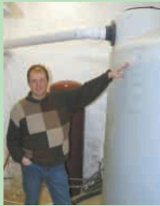
Christian Milaster designed a water storage system that collects rain water from his home's roof. He installed three 2,500-gal. tanks in his basement.
