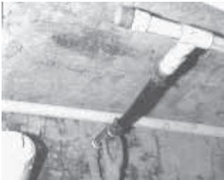
alongside to install a new suction line. Fortunately, the service man who came out to the farm had a simpler solution. He had seen the problem before and just installed a new check valve in the line up by the pump leading down to the old suction line. It solved the problem. The check valve at the bottom of the well just stays open."
