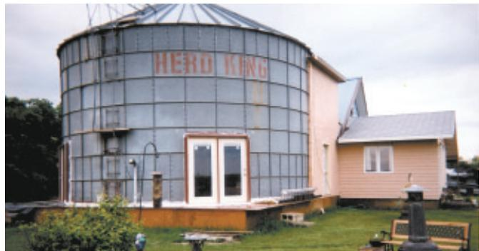
He opened up the end wall of his single story house, and also removed some of the silo’s lower panels to join the two structures.
