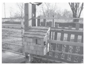
Herron's 24-ft. sliding metal gate is opened by a garage door opener. The opener and other components are housed under a 2-ft. high cover made from cedar shake shingles (above). The entire gate is 24 ft. long, but only 15 ft. of it extends across the driveway.
