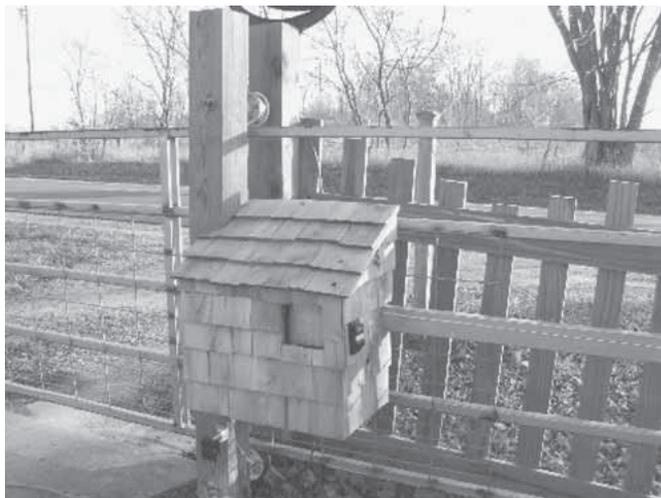
Herron's 24-ft. sliding metal gate is opened by a garage door opener. The opener and other components are housed under a 2-ft. high cover made from cedar shake shingles (above). The entire gate is 24 ft. long, but only 15 ft. of it extends across the driveway.
