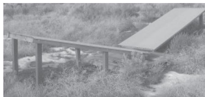
**Man-made water reservoirs for wildlife are refilled automatically when it rains. It's designed to be installed in-ground with a "collector" system over the top to feed water into the tank. It has a 500-gal. capacity and can be transported in a standard pickup bed.**
