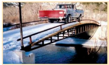
To build vehicle bridges, Ed Stahler uses two spans with bridge planks over top for a 10 Bridges are so light they can be set in place with a front end loader. to 12-ton load rating.
