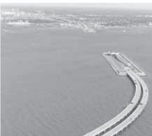
This bridge between Sweden and Denmark "disappears" under the sea so ships can still travel normally overhead.
