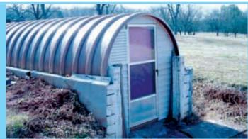
Greenhouse stands on block foundation in trench dug into the side of a hill.
