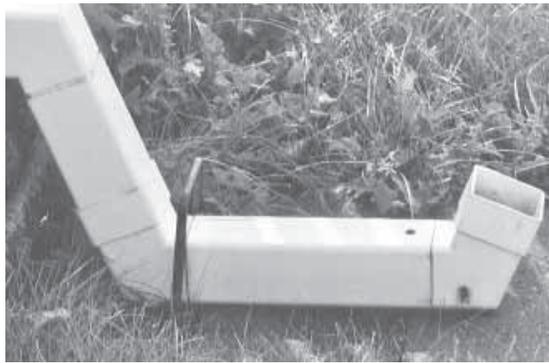
Downspout was made by screwing together three sections of 4-in. sq. PVC tubing. Each section has a 45 degree elbow in it. Holes were drilled into tubing, allowing water to seep out and lose its force.
