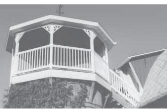
Clarence Douma shortened his silo and then built a wood and fiberglass gazebo on top. He also cut a hole in the barn roof and built a walkway from barn to gazebo.
