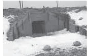
He drove creosote-treated railroad ties into the ground as posts to hold the slats in place.
