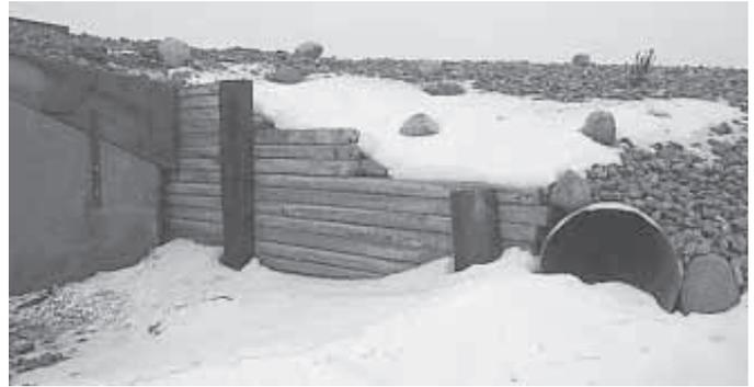
To keep soil from eroding away around a culvert, Blomgren used concrete slats that had been removed while remodeling a hog building.
