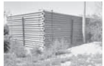
Holes are drilled in center pivot tubes and they're set onto 2 7/8-in. dia. well pipes.
