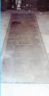
Service pit is equipped with retractable hydraulic floor. When it's not needed, the hydraulic-controlled floor is raised so it's level with shop floor.
