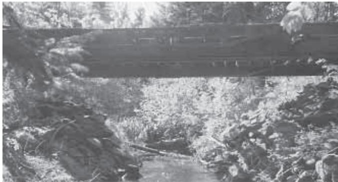
Verleun converted a pair of 40-ft. long, 8-ft. wide semi flatbed trailers into this bridge.
