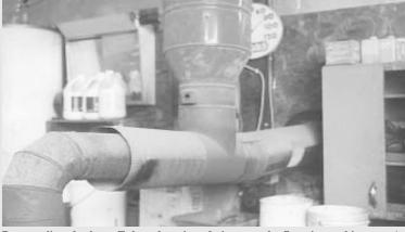
Dunton slipped a large T-shaped section of pipe over the flue pipe on his stove. An aeration fan pulls heated air off the flue pipe and circulates it around his shop.
