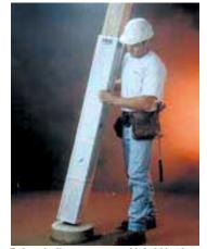
Poly unit slips over post and is held in place by stainless steel lag screws.
