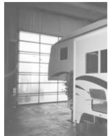
**Thanks to the insulation provided by its triple-layered construction, solar heat captured by the door remains inside.**
