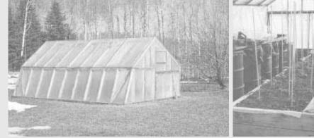
Base of greenhouse is buried 2 ft. in the ground which helps it warm up faster in the spring. The Kuelkens also put 45-gal. barrels along one wall filled with water. Note raised garden beds.
