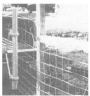
An A-shaped puller is chained to a pickup, tractor or come-along to stretch the fence.
