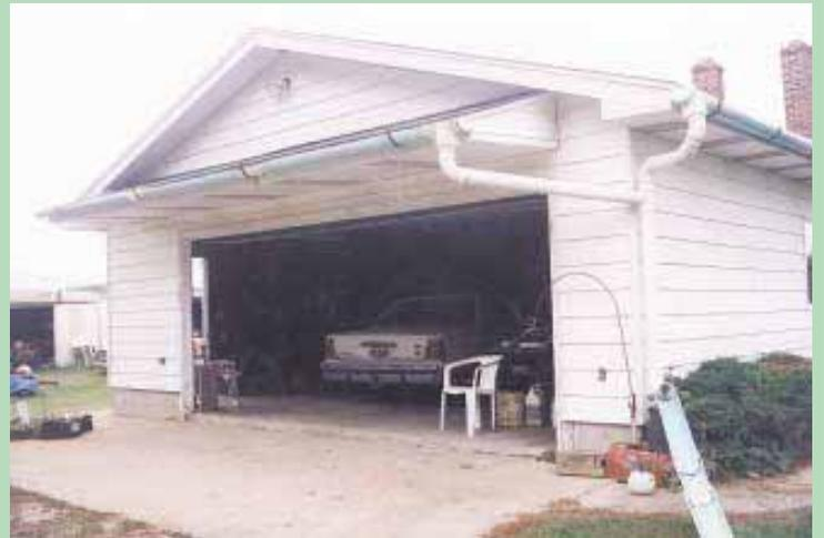
Kaiser used lengths of 6-in. dia., 1/4-in. thick plastic sewer pipe to make eave troughs and down spouts, cutting sections of pipe in half lengthwise and bolting them together.
