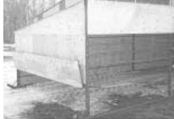
To move the shelter, you flip up the 20-in. flap on the end and simply tow it away.
