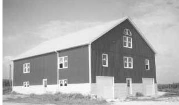
The barn as it looks today. The crumbling old foundation was replaced with new concrete and the barn was sided and roofed with steel siding.
